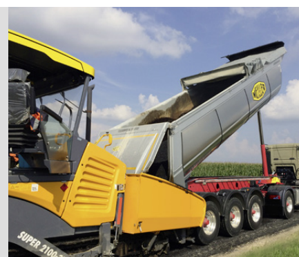
Tar surface finishing: With the tarpaulin closed, the asphalt retains its required temperature.
